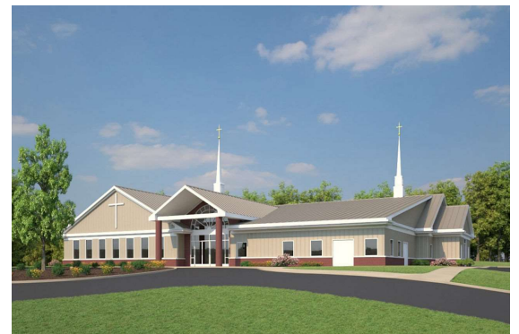
Prospective Church Building
